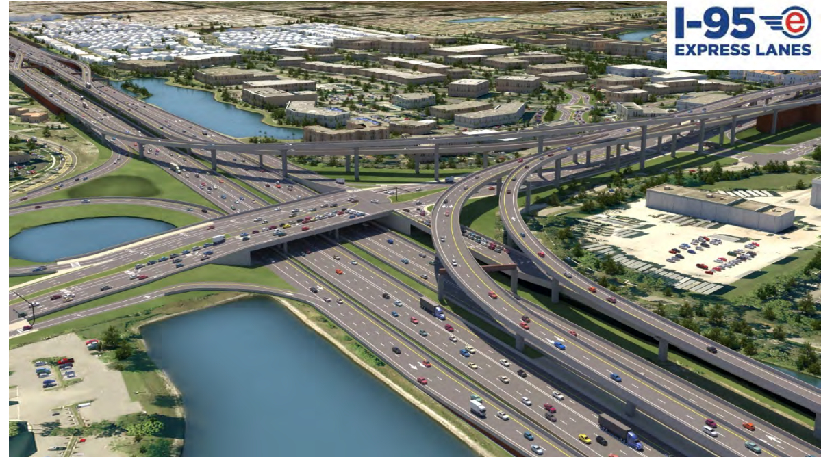
I-95 from SW 10 th Street to Hillsboro Boulevard PD&E Study
