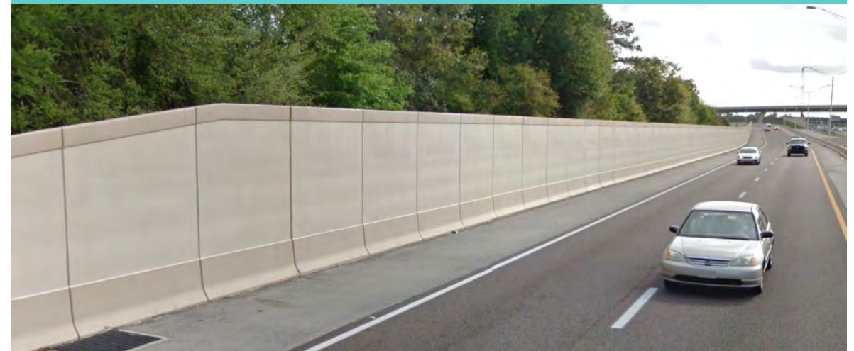
Example shoulder-mounted noise wall
